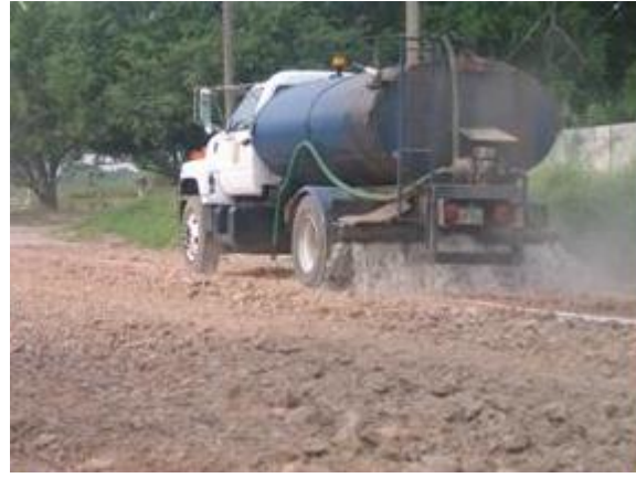
The water truck applies the product/water mix over the road area after the first ripping pass of the grader.
