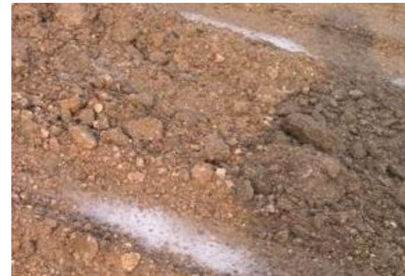
More of the road surface is treated, then ripped again and again.
