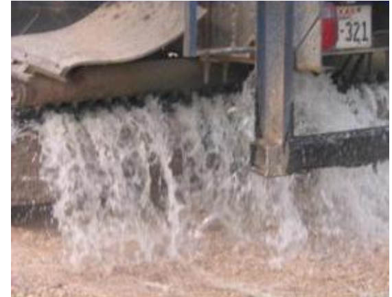
The water truck applies the product/water mix over the road area after the first ripping pass of the grader.
