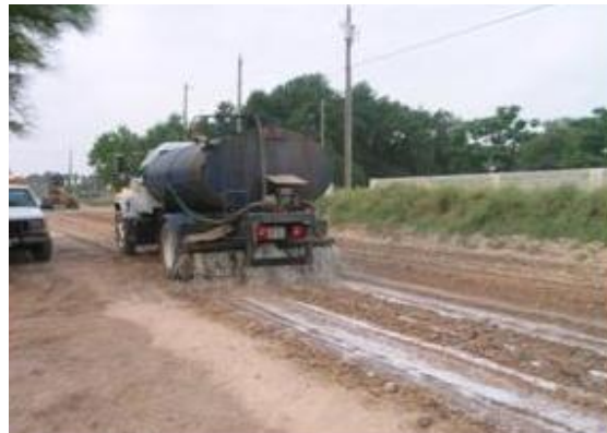
More of the road surface is treated, then ripped again and again.
